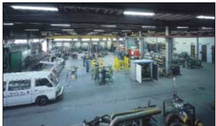
M&R Stations Manufacturing Plant, Essen, Belgium
