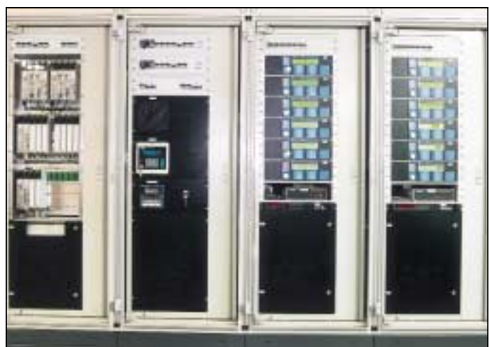
Redundant orifice metering 4,700,000 m 3 /h at 60 bar
